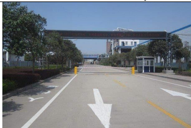
Factory production area
